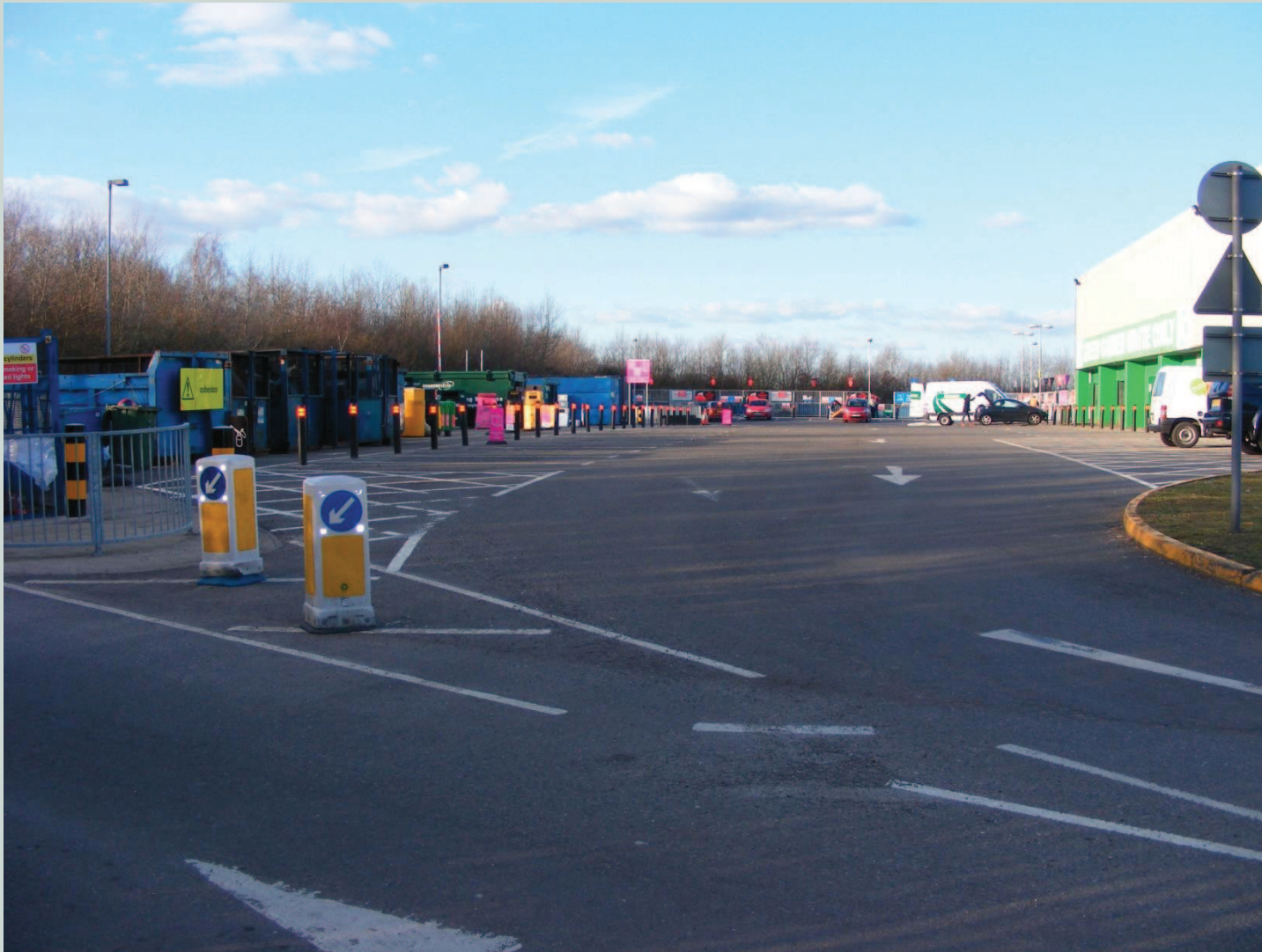
Fig 2 : View of CRC and WTS looking north within the site
