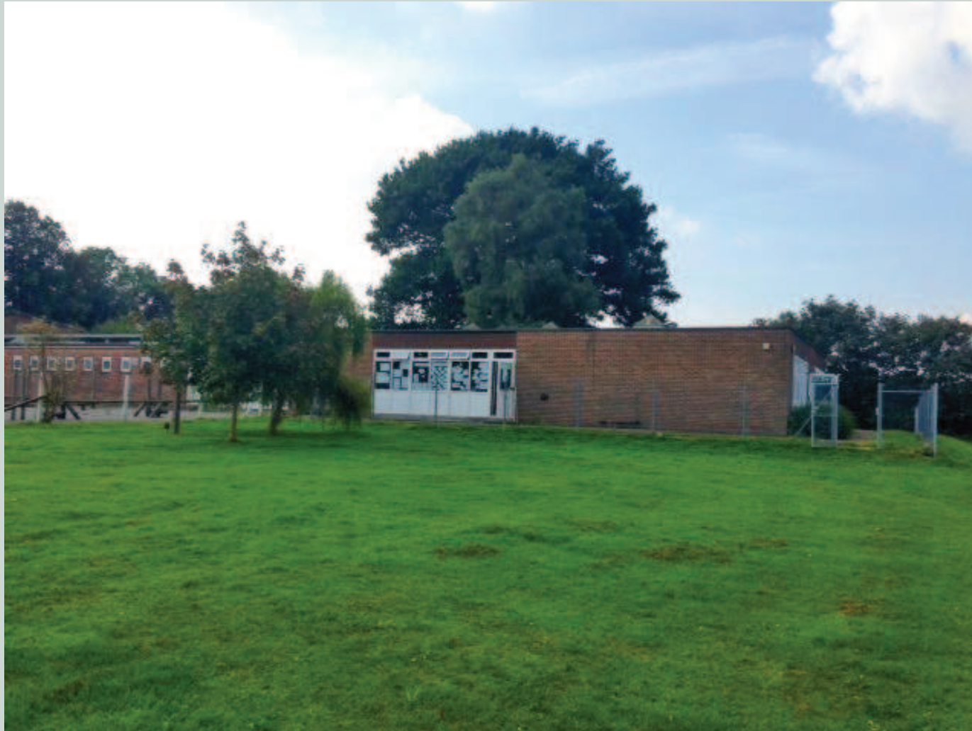
Fig 1 : Site of proposed extension looking South
